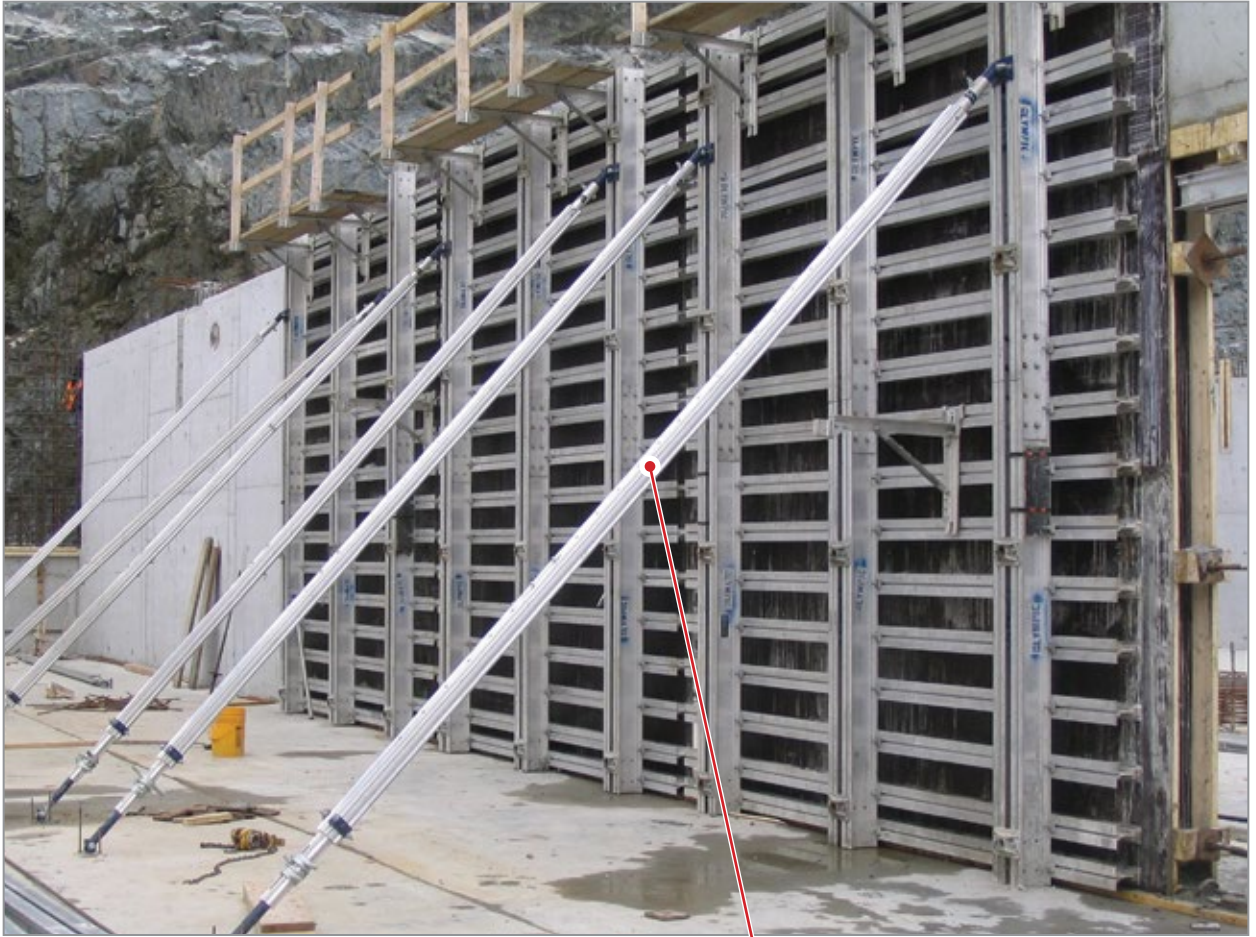
Post shores transformed into 30' long Aluminum Push and Pull Braces
